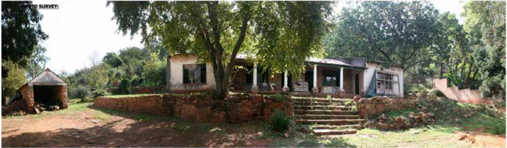
PHOTO SURVEY: MAIN BUILDING A - SOUTH ELEVATION (2011): REFER SITE PLAN P31
